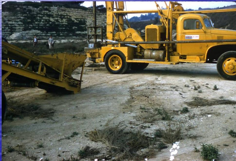
Around 1960 several southland geologists began using large diameter bucket auger excavations to assess complex geologic conditions. This became the preferred method of site exploration over the following decade.
